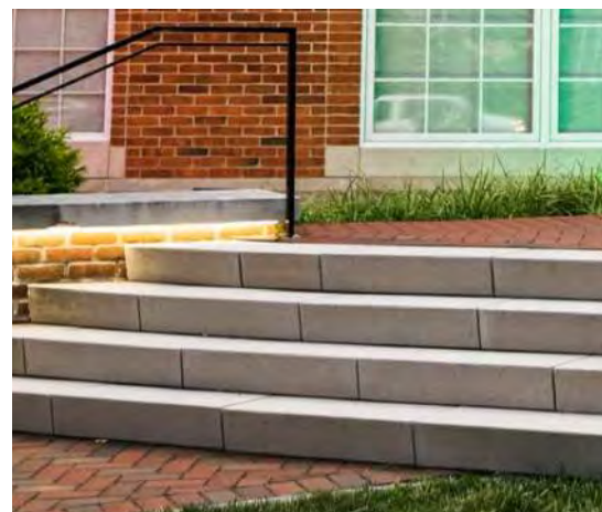
Cast Stone Stairs
