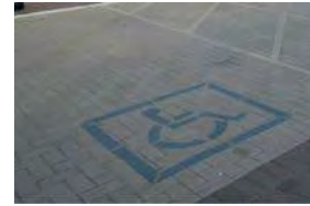
PAVER TYPE (6) Belden Brick Company ADA Blue Kiln Fired on City Line Landmark Gray Pavers (ADA Markings)
