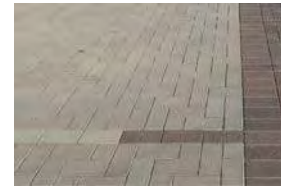
PAVER TYPE (5) Belden Brick Company City Line Lighthouse Gray (Parking Striping) w/ Seinna 3 Paver Stripe End
